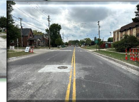
Longvale-Woodbrook & Lee Road Reconstruction in Progress
